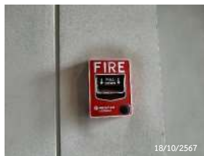
Fire Alarm Manual Station
